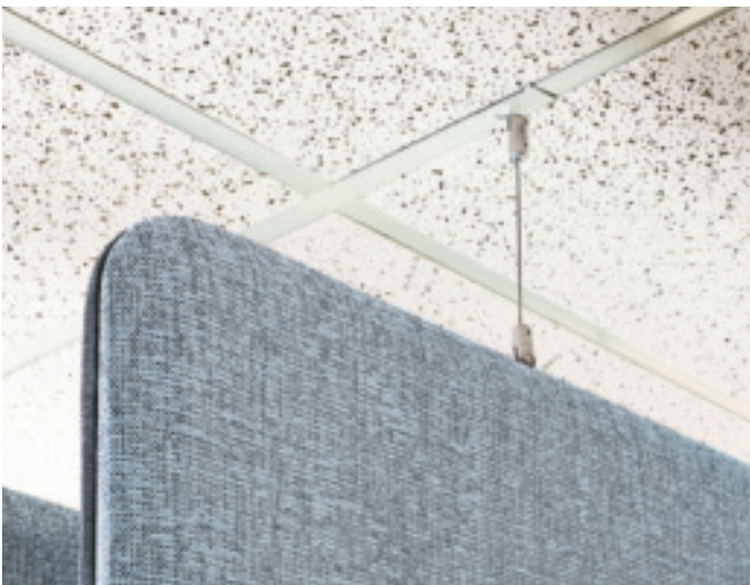
Drop Ceiling Vertically Suspended Baffles Using Cables
